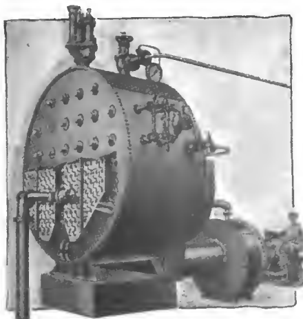
Fig. 3—Experimental 500-hp. flameless surface-combustion steam boiler tried in England and Germany. First type tried
